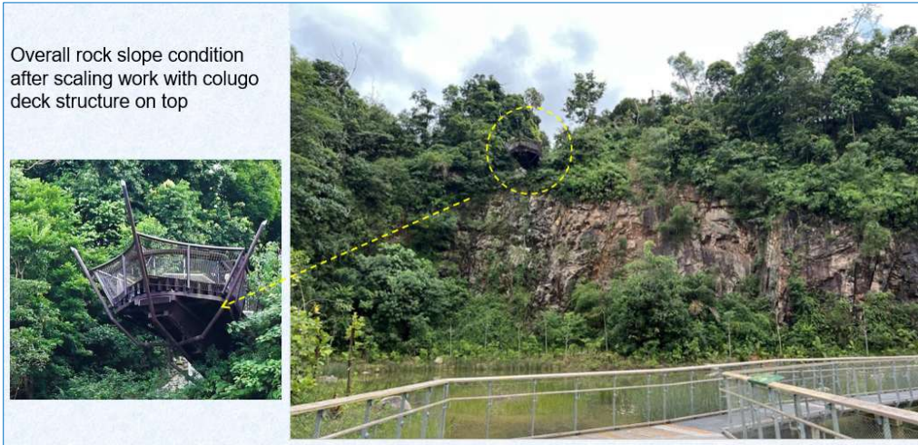
Fig. 9. Overall rock slope condition after scaling work with colugo deck structure on top (Project 1)
