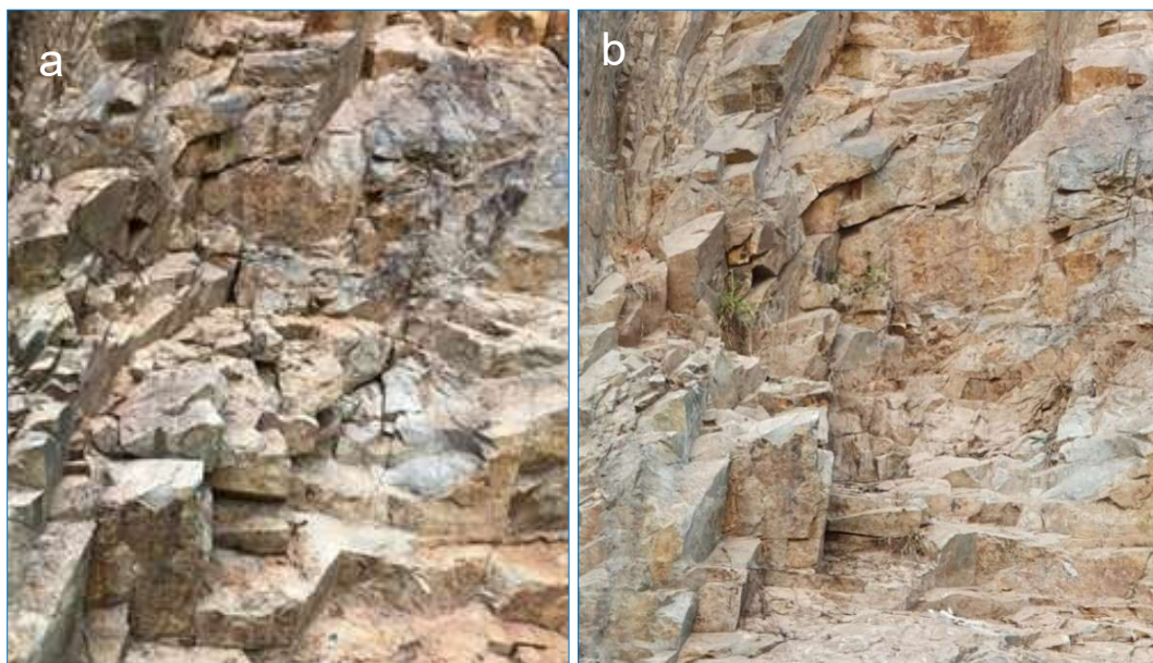
Fig. 8. Comparison of rock slope condition at some selected locations (Project 1): a) before scaling work and b) after scaling work
