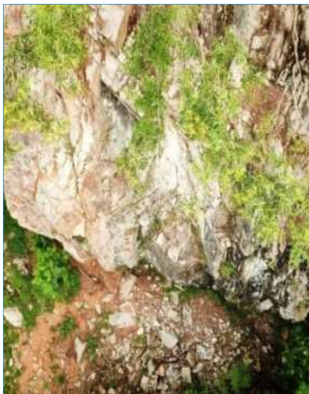
Fig. 12. White-coloured loose residual soil falling from slope top (Weathering effect-controlled rock slope failure)
