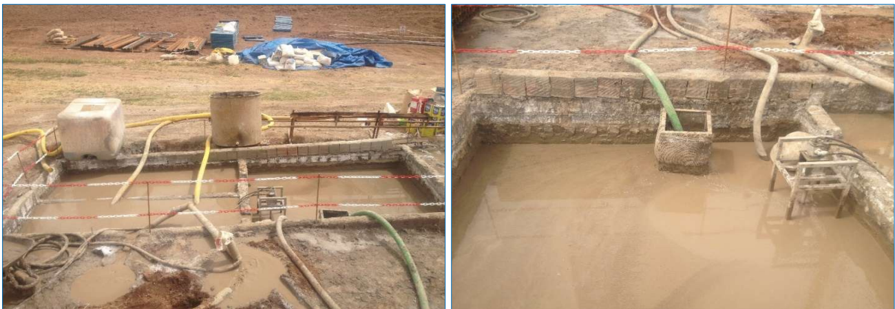
Fig. 7. Ensuring movement of mud continuously mixed through a mixer placed in the mud pits
