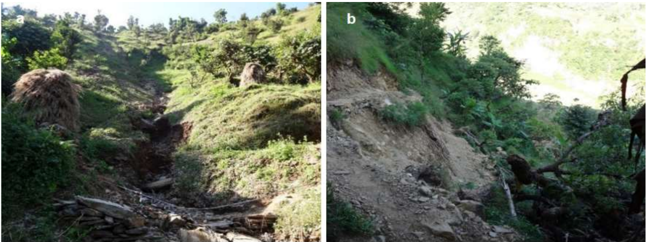
Fig. 16. Damages during rainfall in Dhami Tok; (a) Gully erosion by seasonal nala and (b) the ground fissures in the agricultural fields at Dhanari
