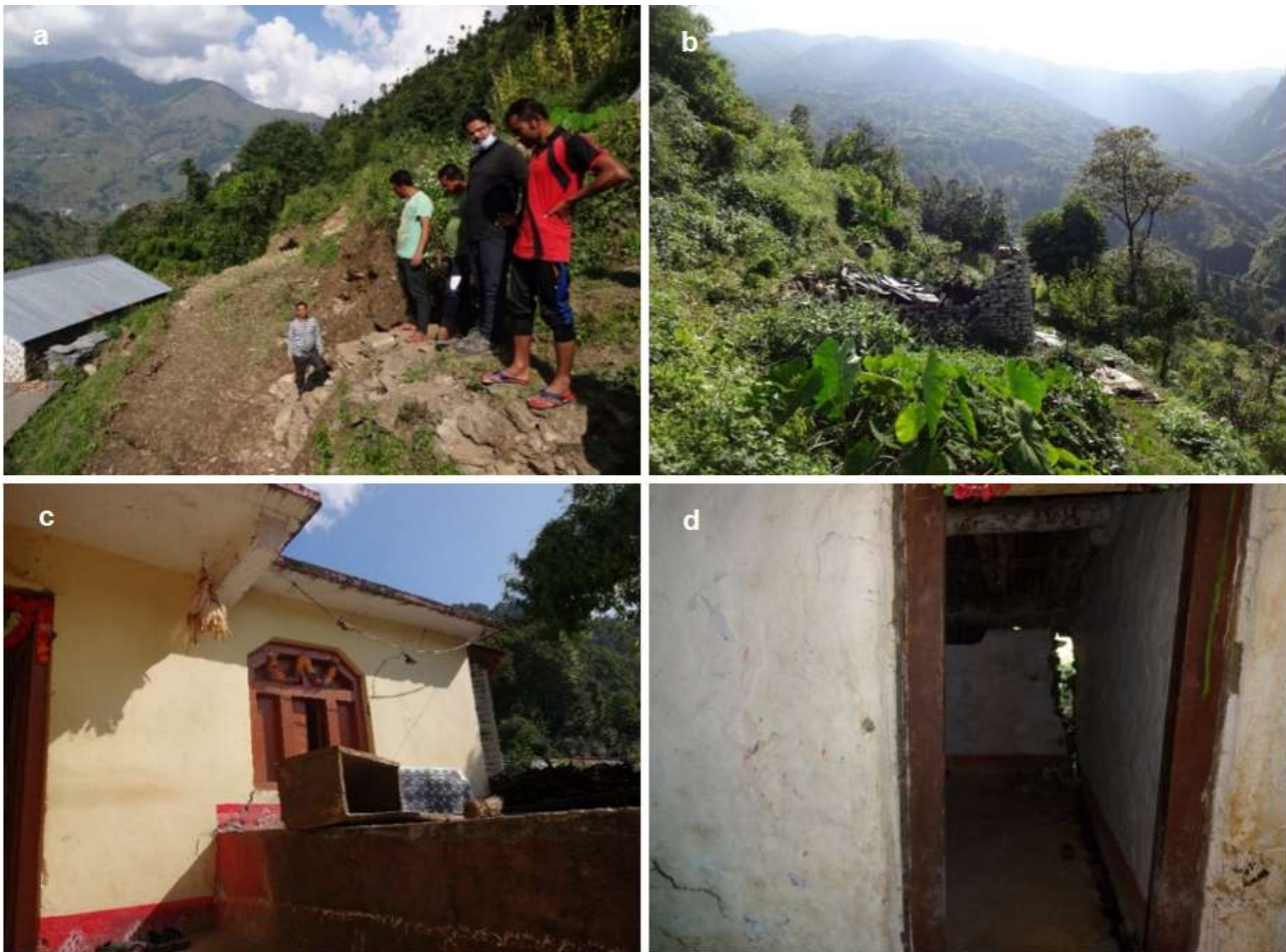
Fig. 7. Ground subsidence related damages in the Malupati Village; (a) ground fissure in agricultural fields, (b) collapsed a house, (c) crack in a house and (d) detached back side wall of a house
