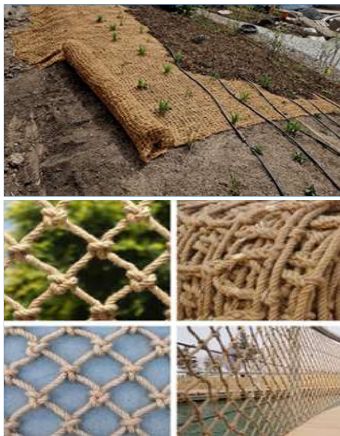
Fig. 26. Jute and coir net used for slope cover in bioengineering works
