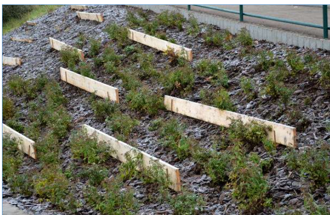
Fig. 34. Palisade vegetated system (using personal device)
