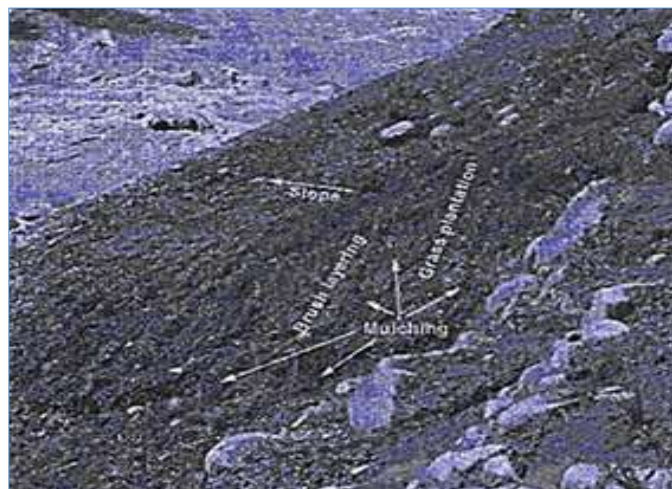
Fig. 42. Mulching on the slope (using open source)
