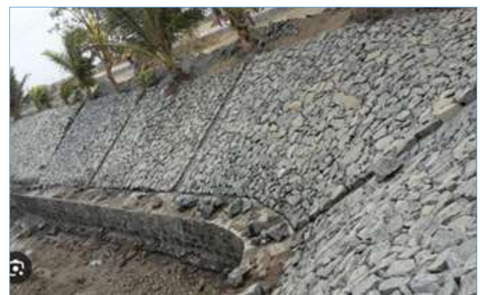
Fig. 25. Stone pitching at the face of water stream areas (using personal device)
