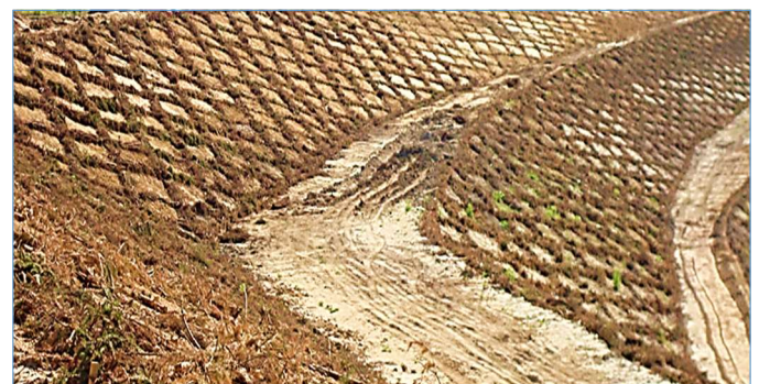
Fig. 36. Fence implemented as a bioengineering system (using personal device)
