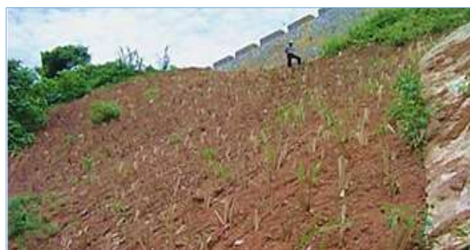
Fig. 31. Diagonal line of grass plantation (personal device)
