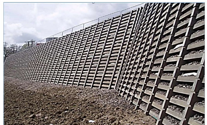
Fig. 14. Crib wall at the sloppy different materials (adopted from open source)
