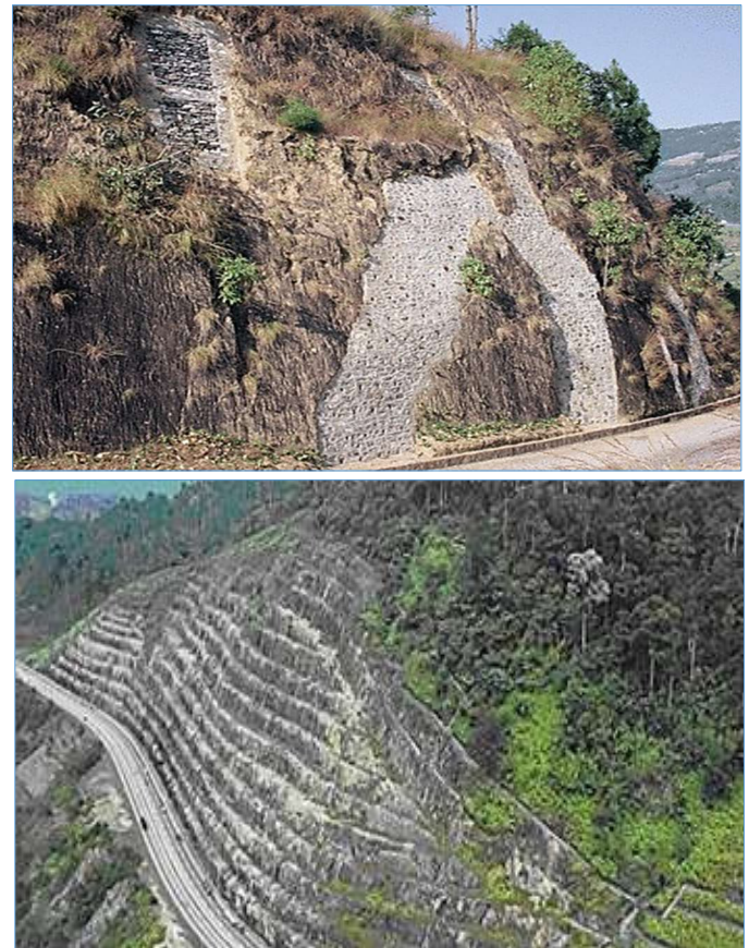
Fig. 24. Roadside slope protection by wattle fence
