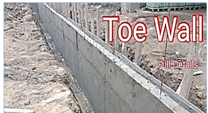
Fig. 18. Toe wall at the agricultural lands (adopted from open source)
