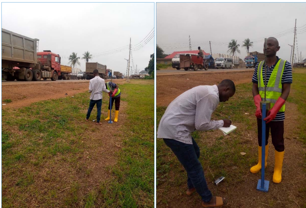
Fig.5. DCPT Field Survey carried out along Akure–Owo Highway at different locations
